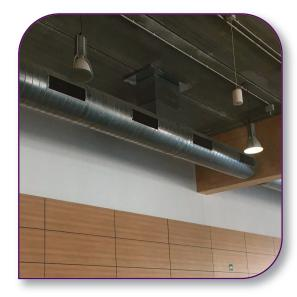
CMC+SD (T) M9006 dim. LxH, constructed from galvanised steel paint in grey M9006 with flap damper from steel SD, visible fixing screws (T).
